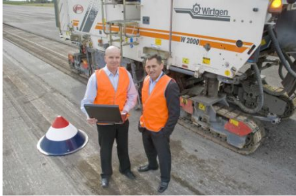
David Sammut and Patrick Archer, of Cedar Woods, at Williams Landing as construction commences
